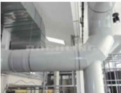
Polystone® PPs grey Ventilation plant
