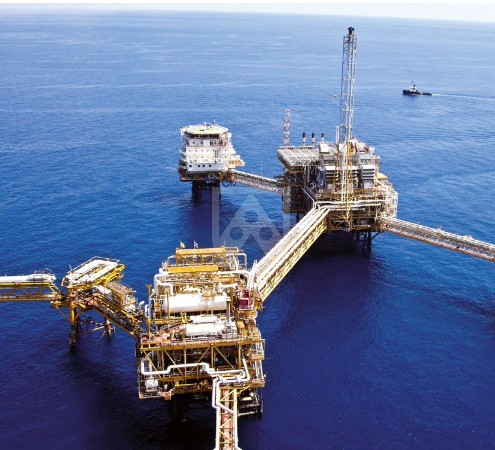
陆上/海上工程 Onshore/offshore engineering
