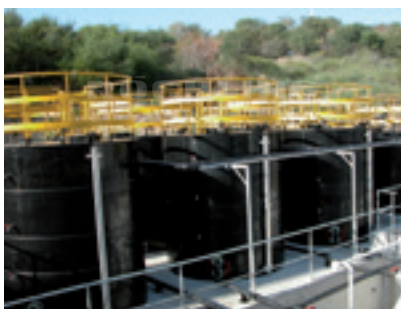
Polystone® G black B 100-RC 盐酸储液罐
